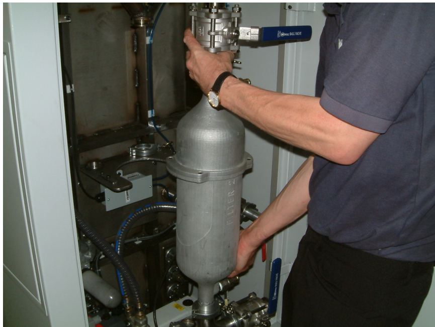
Fig FILTER 2 REMOVAL Note the valves in the closed position
